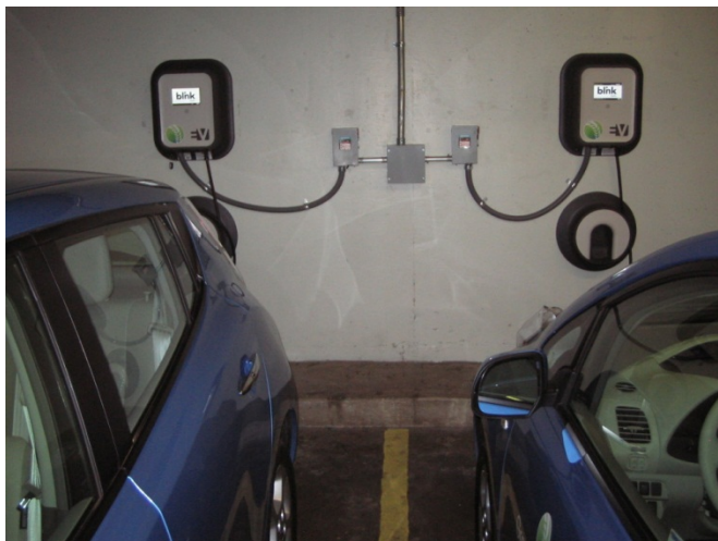
Ecotality chargers in Waikiki hotel parking garage.
