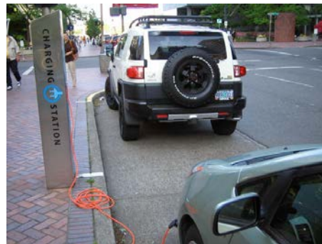
On-street parallel EV parking space features pedestal-mounted charger.
