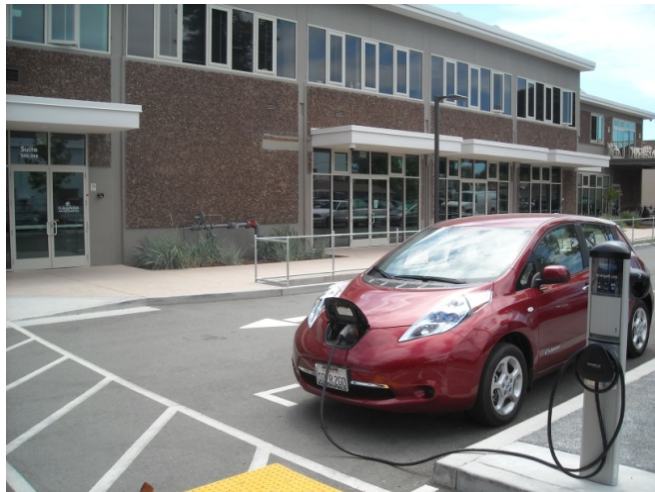
Charger installed for parallel EV parking in lot near pathway to building entrance.
