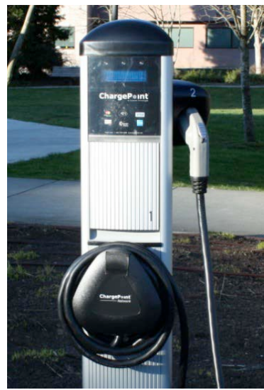
Coulomb charger featuring Level 1 and Level 2 charging.
