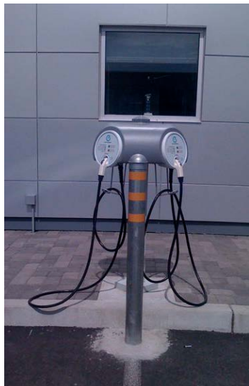
AeroVironment charger with dual port capability.
