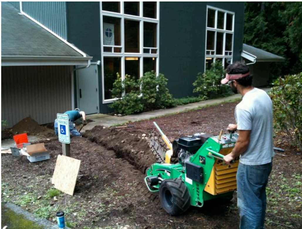
Workers dig conduit trench from electrical supply point to EV charger location.
