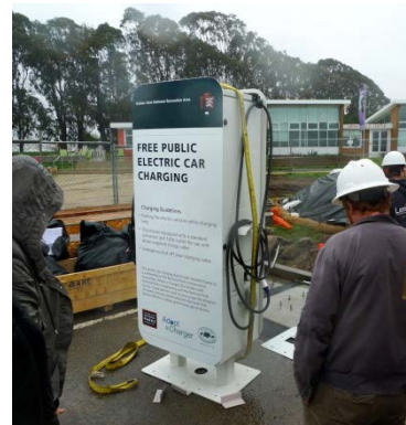
Adopt a Charger installation, Crissy Field, San Francisco. Photo courtesy of Marc Geller
