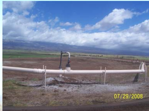
Gas Collection System Distribution Line ~ 7,000 feet of pipeline
