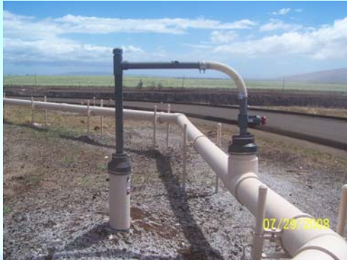
47 Gas Collection System Vertical Well Heads ~ 30-120 foot depth
