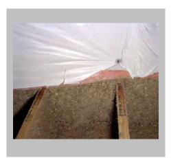
disaggregating into fibers (fiberization). The simplest use is blowing or pouring loose-fill cellulose into the attic space to provide about R-3.7 per inch. To reduce flammability and deter
