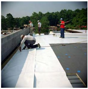
Roofing membranes are typically available in shades of black, gray or white. The reflectance and emittance of roofing membranes have a significant impact on the air-conditioning load of a building. Products with a high reflectance and emittance are recommended. Light-colored membranes may cost more, but the additional cost is usually balanced out by reduction in thickness of insulation required to comply with code.
