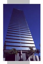
Windows are the critical element in office solar control. Proper orientation and exterior shading are the preferred approach. Otherwise, glazing with low solar transmission is appropriate (but also remember light transmission for daylighting). See the Energy-Efficient Windows Guidelines for recommendations.
