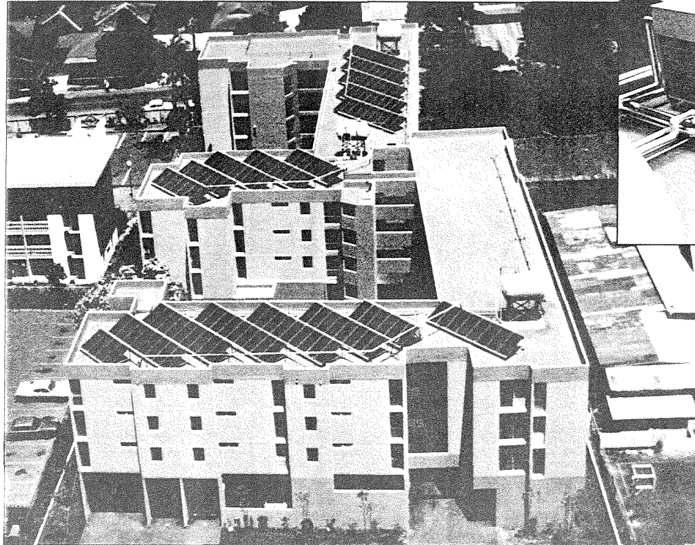
H.1 Banyan Street Manor Condominiums, 1977. Solar collectors for water heating were designed as an integral part of the building. Architects: Milton Sher & Associates. Solar design and photograph: Mike Bean.
