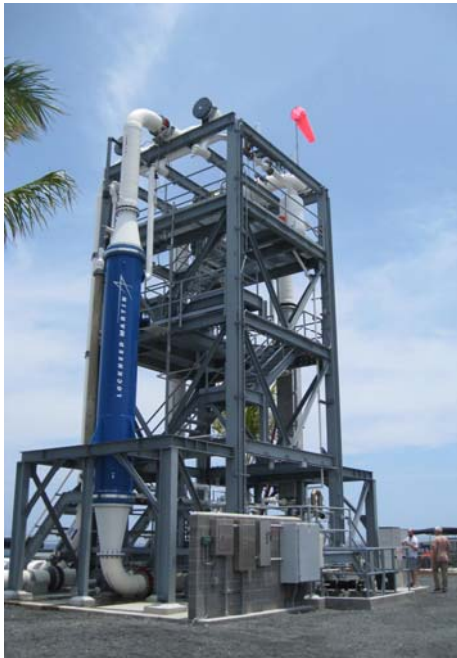
Figure 4: Heat exchanger test tower operated by Makai Ocean Engineering at NELHA.
