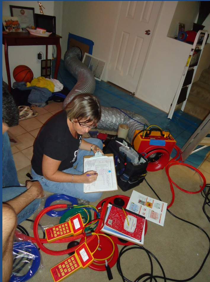
Duct testing in an occupied home
