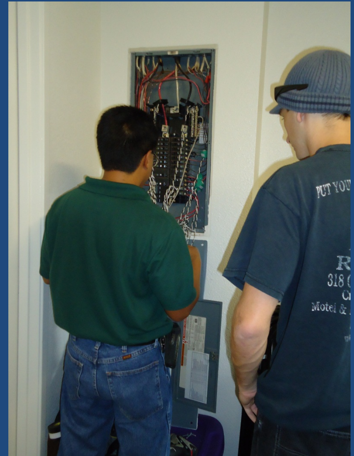
Installing current transducers
