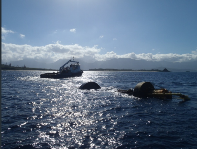
WEC Device Being Delivered On-Site
