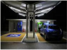
OKINAWA EV Charging Spot
