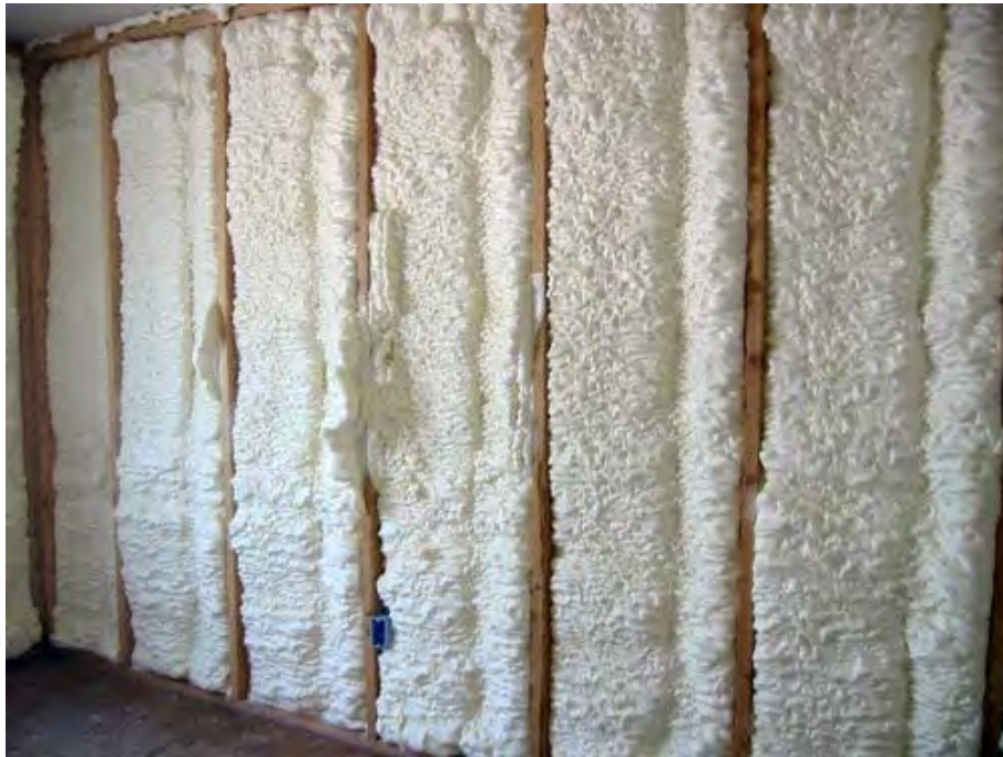
Source: DOE/NREL PIX13528
