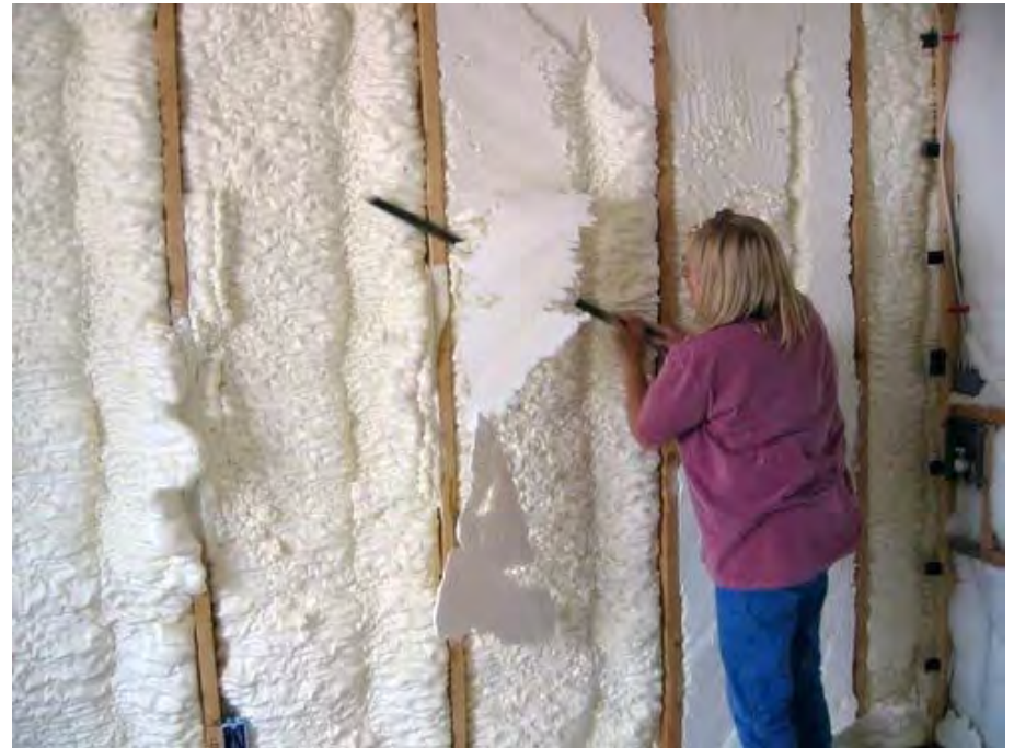
Source: DOE/NREL PIX11530
