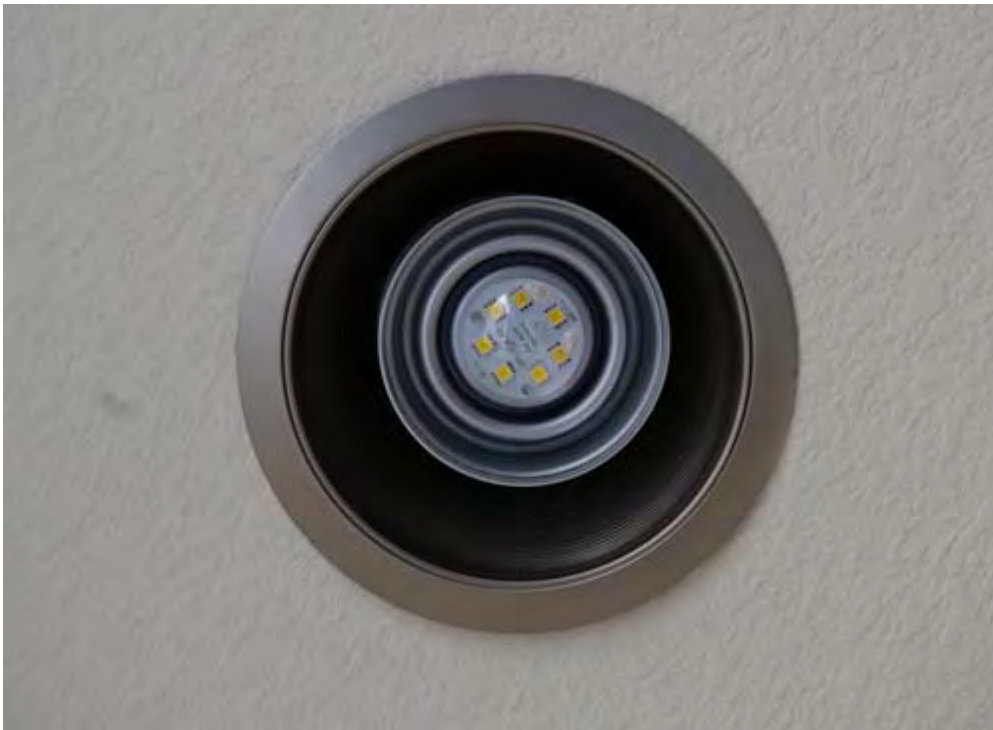
Source: DOE/NREL PIX20310
