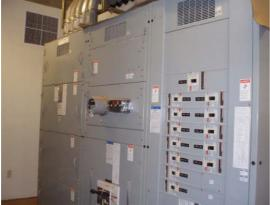
The following picture shows a switchboard with fuses installed instead of breakers. Older buildings have this type of design.
