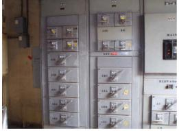
• The following photos shows a Distribution Panel which a majority of condominiums have which consist of molded case breakers for specific areas and panels. This would be the other equipment that any EV charging stations would get power from since a specific panel for EV charging stations could be installed from this point in the electrical system.
