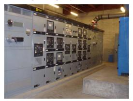
• The following picture is that of a switchboard which has breakers that are bolted onto the equipment and to replace breakers. The entire electrical system would need to be turned off in order to unbolt breakers safely. This is the majority of equipment installed in buildings due to costing. The same rule applies for the switchboard as to HECO's responsibility and the
