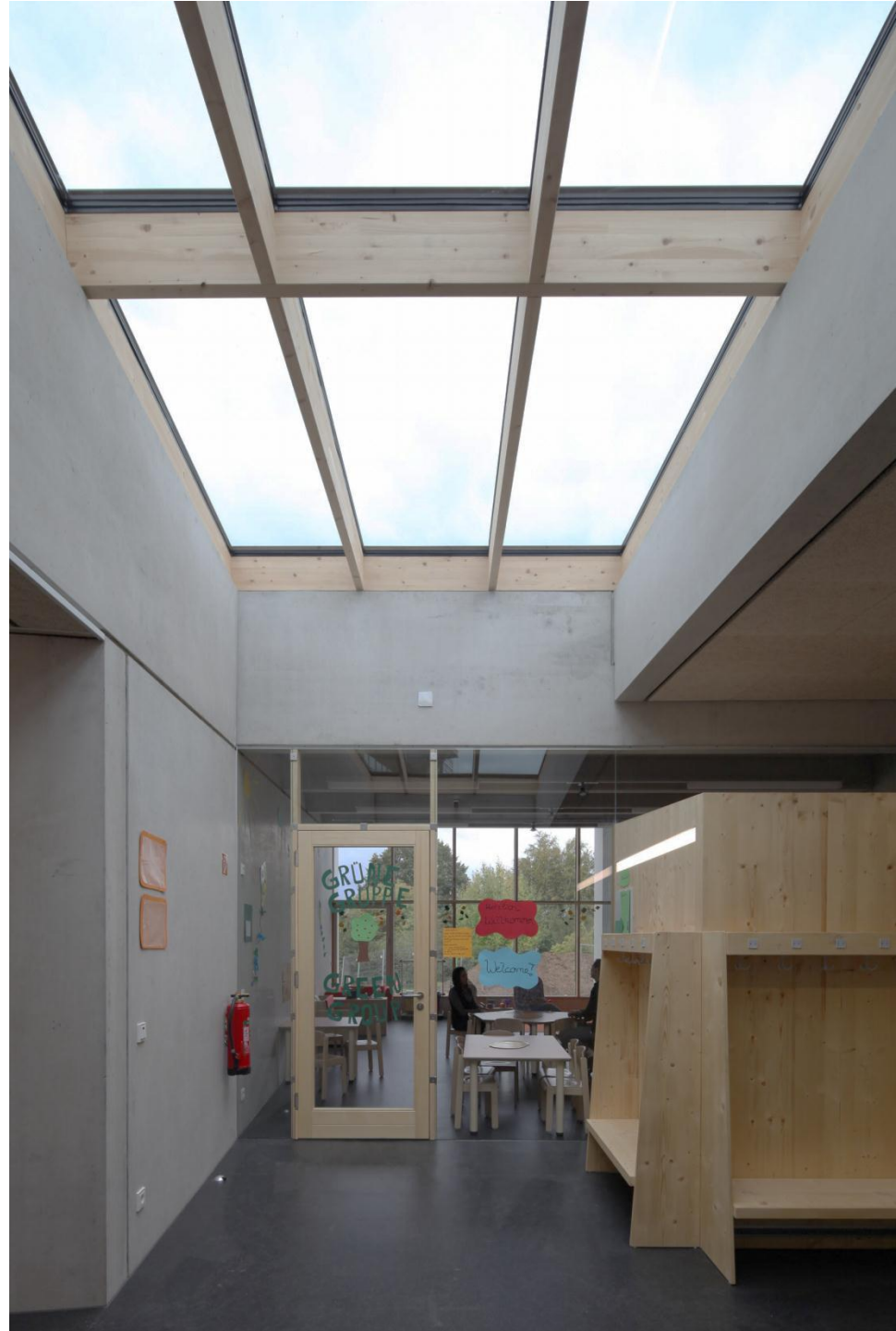
the standards help shape the building's architectural form, being a solid mass prefab concrete building, which is softened through the use of wood and light perforations.
