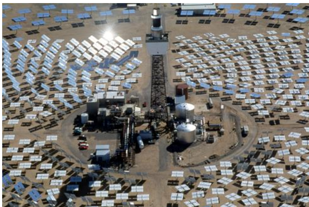
Figure 2-40. Operating Solar Power Facility in Spain
