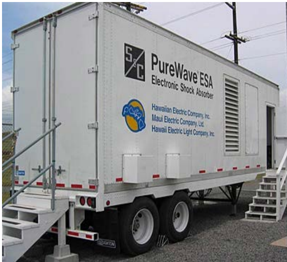
Figure 2-67. Ultra Capacitor Installation
