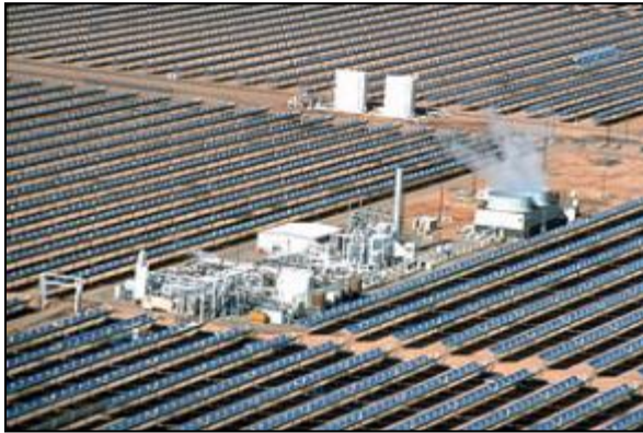
Figure 2-38. Parabolic Trough Solar Farm with High-Temperature Solar Collectors and Support Facilities, Cooling Towers, White Water Tanks, and Generation Equipment (Source: DOE-EERE 2013b)
