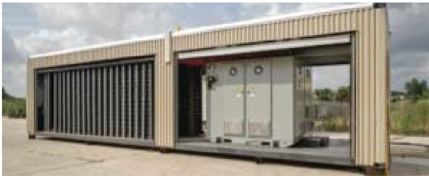
Battery storage, such as this unit by XTreme Power, can mitigate the impact of intermittent renewables on the grid.
