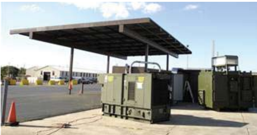
This hydrogen fueling station, partially powered by PV at Hickam Air Force Base, exemplifies DOD's interest in renewable fuels
