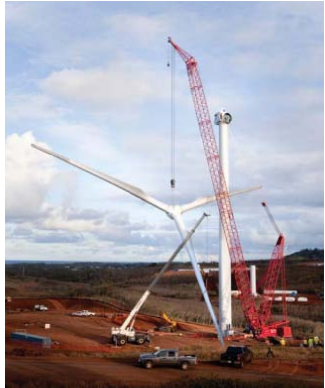
The Kahuku wind farm consists of twelve 2.5-MW Clipper Liberty wind turbines and a 10-MWh Xtreme Power battery storage system.
