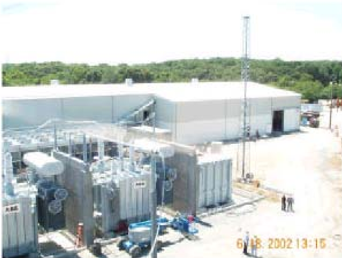
VSC HVDC Converter Station (background) and Transformers (foreground)
