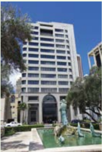
State Office Tower (SOT) Certified Prestigious LEED Gold.
