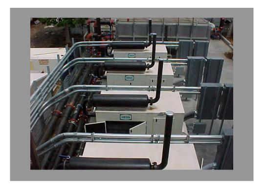
The Pohai Nani assisted living facility in Kaneohe uses one 100-kW propane engine generator (made by Hess Microgen) that provides heat for two 10-ton absorption chillers, domestic hot water and a swimming pool.
