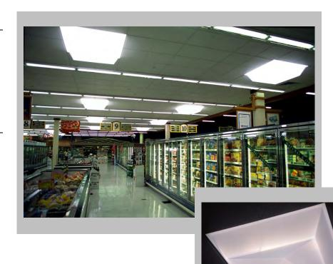
The Better Brands warehouse on Oahu employs a similar skylight system with integrated light wells, which also includes electric lighting. These units contain six 4-ft T-5 fluorescent lamps mounted behind the diffuser at the bottom of the light well. These lamps can be controlled in several steps to supplement daylight or provide nighttime illumination.
