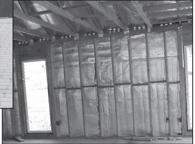
Above: Astro-E was draped from the rafters and nailed outside the studs. The radiant barrier reflects the sun's heat, helping the home to be comfortable without air conditioning.
