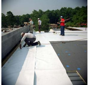
Roofing membranes are typically available in shades of black, gray or white. The reflectance and emittance of roofing membranes have a significant impact on the air-conditioning load of a building. Products with a high reflectance and emittance are recommended. Light-colored membranes may cost more, but the additional cost is usually balanced out by reduction in thickness of insulation required to comply with code.
