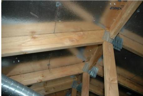
*Radiant barrier under the roof*
