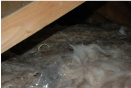
*R-30 batt insulation on attic floor*
