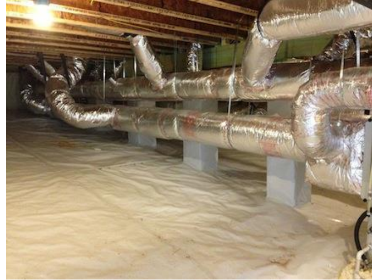
Insulated crawlspace ducts. https://www.energyvanguard.com/blog/the-invisible-problem-with-duct-insulation/
