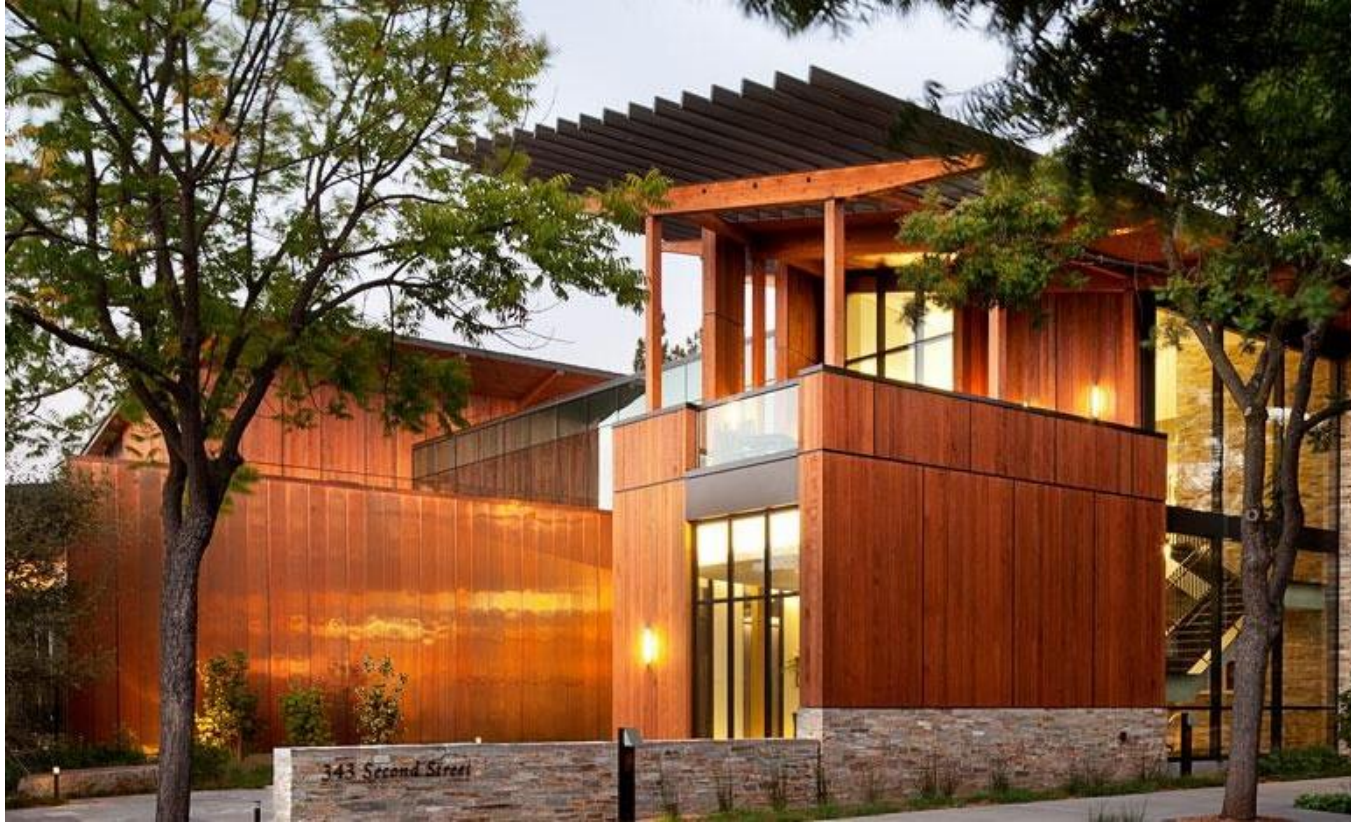
Living Building Challenge™ Net Zero Energy Building Certified David & Lucile Packard Foundation Headquarters Los Altos, California
