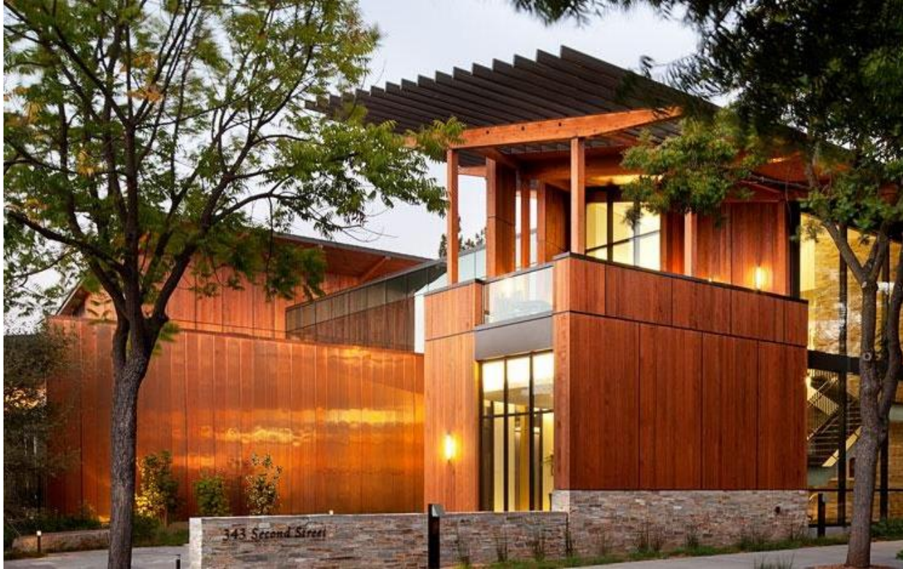
Living Building Challenge™ Net Zero Energy Building Certified David & Lucile Packard Foundation Headquarters Los Altos, California
