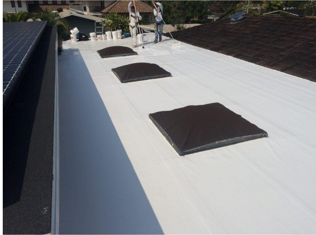
Cool roof - liquid applied example
