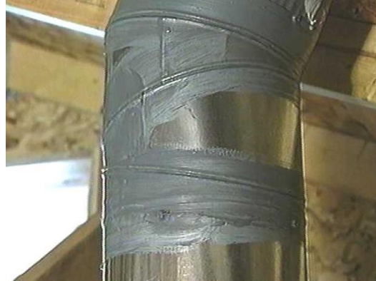
Duct sealing & fastening
