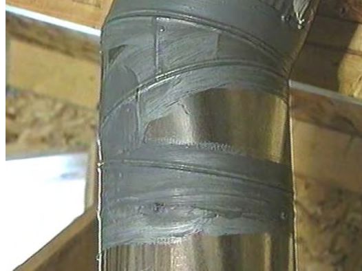
Duct sealing & fastening
