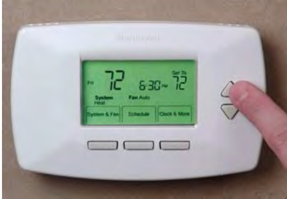
Programmable thermostat
