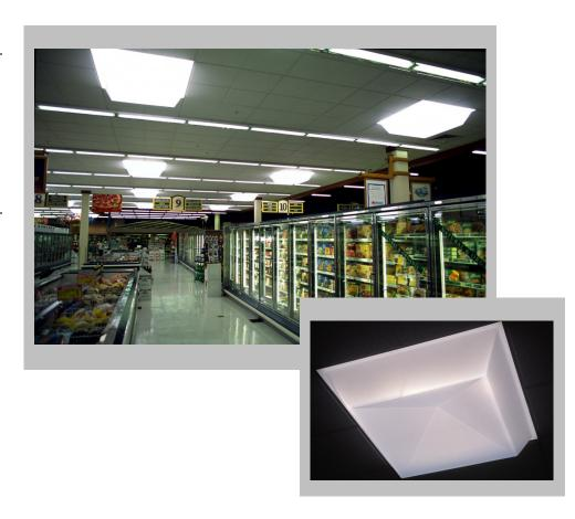
The Better Brands warehouse on Oahu employs a similar skylight system with integrated light wells, which also includes electric lighting. These units contain six 4-ft T-5 fluorescent lamps mounted behind the diffuser at the bottom of the light well. These lamps can be controlled in several steps to supplement daylight or provide nighttime illumination.
