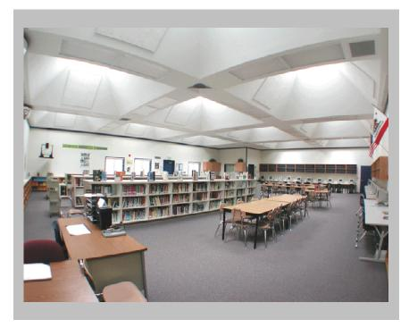
Figure 3-3. Deeply coffered ceiling helps to diffuse light from skylights. White ceilings and walls help reflect light into the space. Photo: SunOptics.
