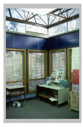
Figure 3-4. Horizontal blinds allow control of brightness from lower view windows. Note that high clerestory windows have no blinds so that daylight can reach deep into the space. Photo: Barbara Erwine.
