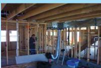
Leakage ≤ 4 cfm/100 ft<sup>2</sup>
