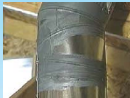
Duct sealing
