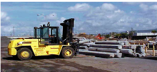
Concrete pile cutoffs were collected and hauled to a Department of Transportation site for reuse/recycling.
