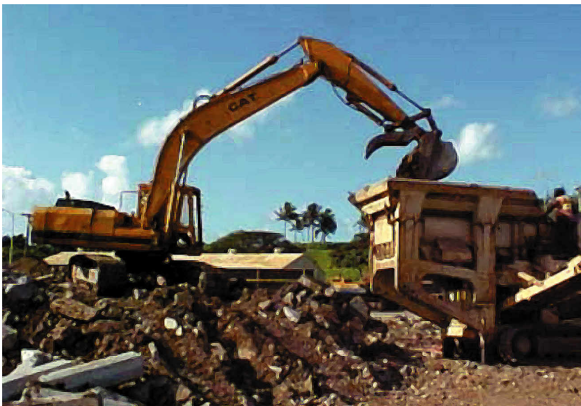
Crushing concrete waste for reuse onsite as aggregate.
