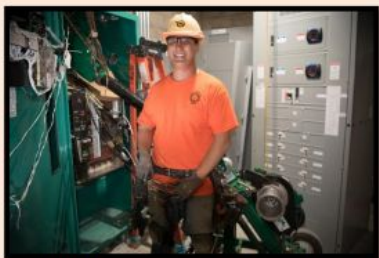
Pulling feeder conductors in an electrical room.
