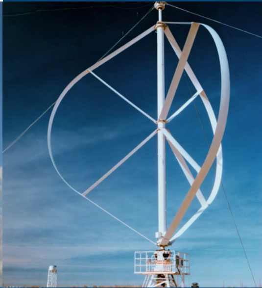
Vertical-axis: Spins like a top.
