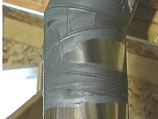
Duct sealing & fastening
