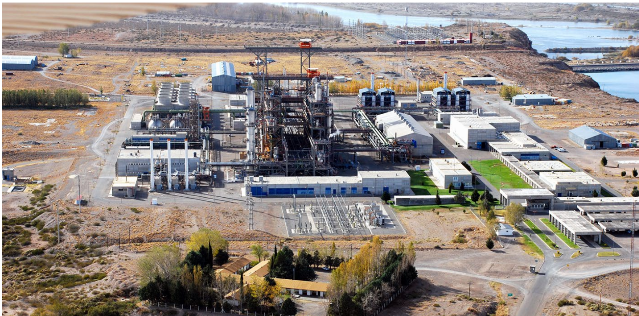
Figure 22. Image of Ammonia Processing Facility 123
